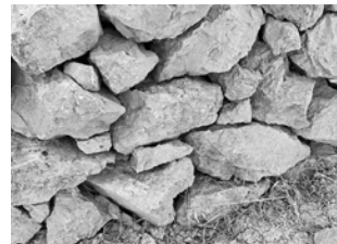
Stone wall used for experiment 2, Moulay Bouchta, 2018.
